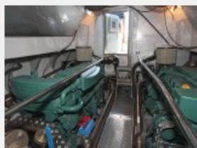
Seaward Nelson 35 Pilot Boat Engine Room
